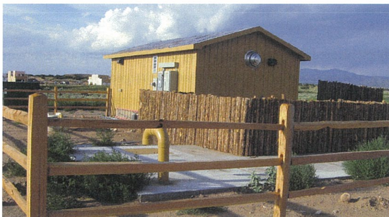
“ Esber ”, Oshara’s Wastewater Reclamation Facility, 2007
